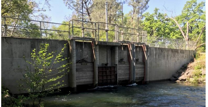
Photograph 1: Lindo Channel Gates
