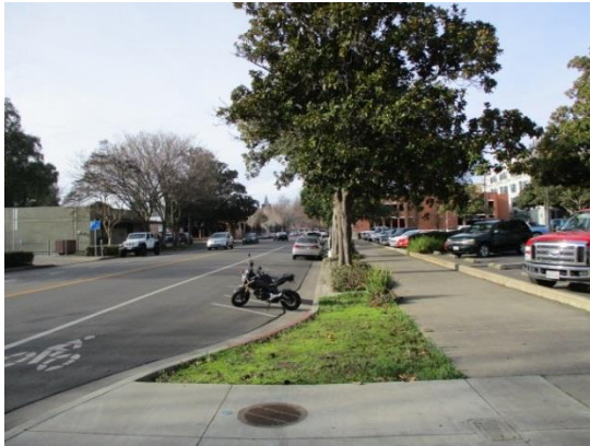
Photograph 1. Potential for a green street project area. Corner of Salem Street and West 5 th Street facing northwest.
