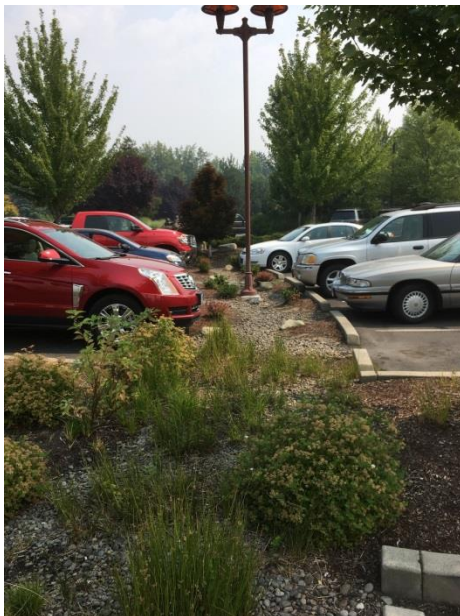
Photograph 3. Example of a bioswale in an Oregon parking lot.
